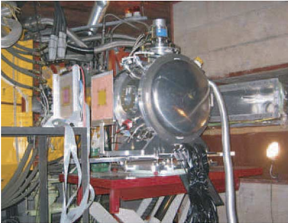
Fig. 10. Direct measurement of heat load in the KEK 12 GeV PS.
